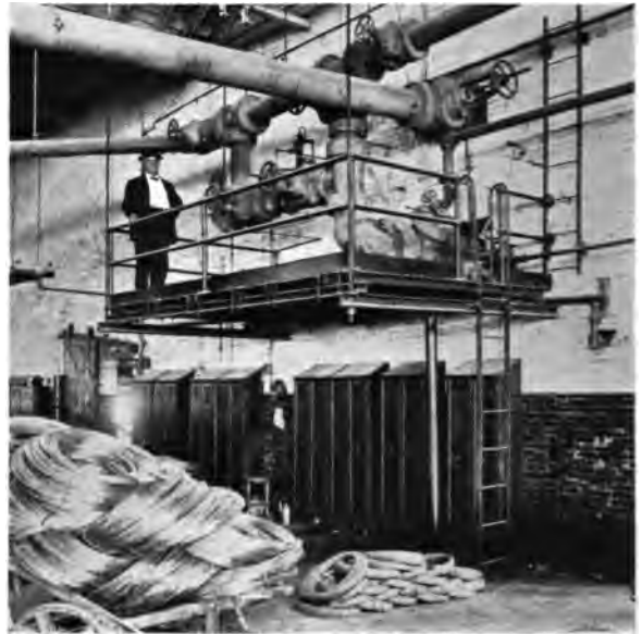
Fig. 2. Standard Railing and Toe-board for Overhead Platform.†
